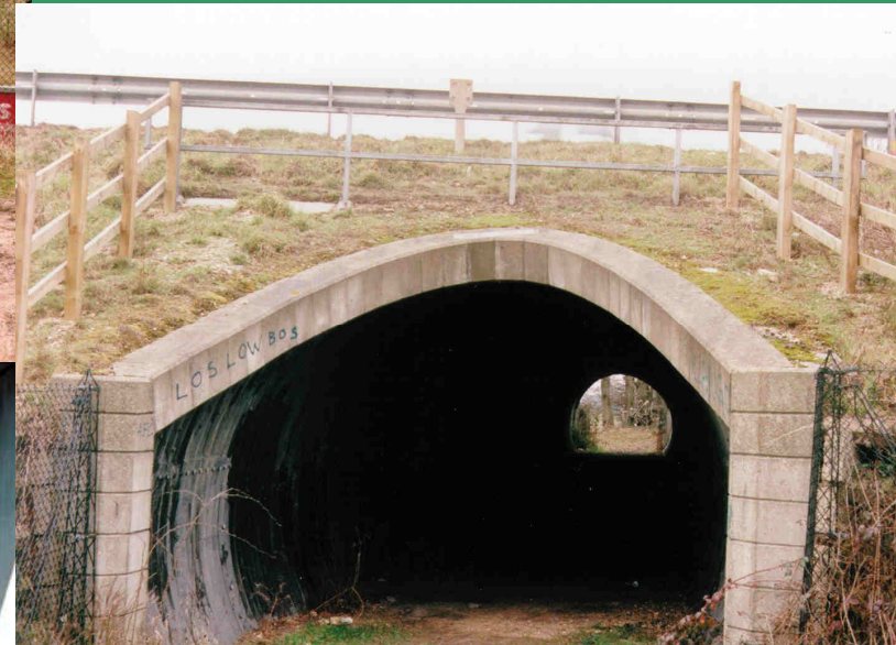
M25 Bridge & tunnel used by fallow and muntjac
